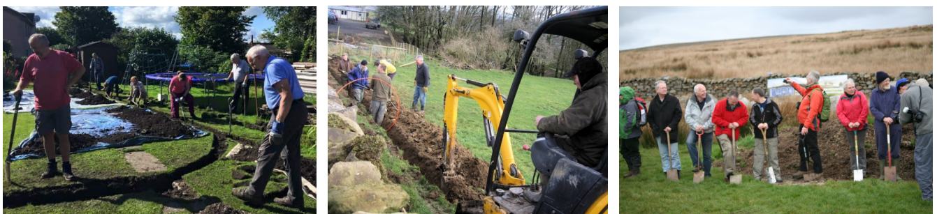
Figure 3.1: Community involvement in laying out fiber through the farmland.
